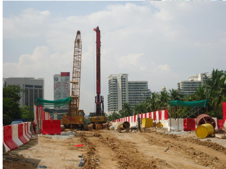
Project : The Construction And Completion of Facilities Works (Package A) For The Kelana Jaya (KLJ) Line Extension Project - Bored Piling Works
