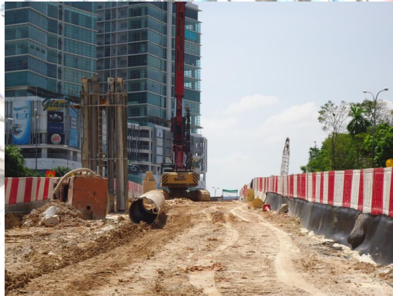
Project : The Construction And Completion of Facilities Works (Package A) For The Kelana Jaya (KLJ) Line Extension Project - Bored Piling Works
