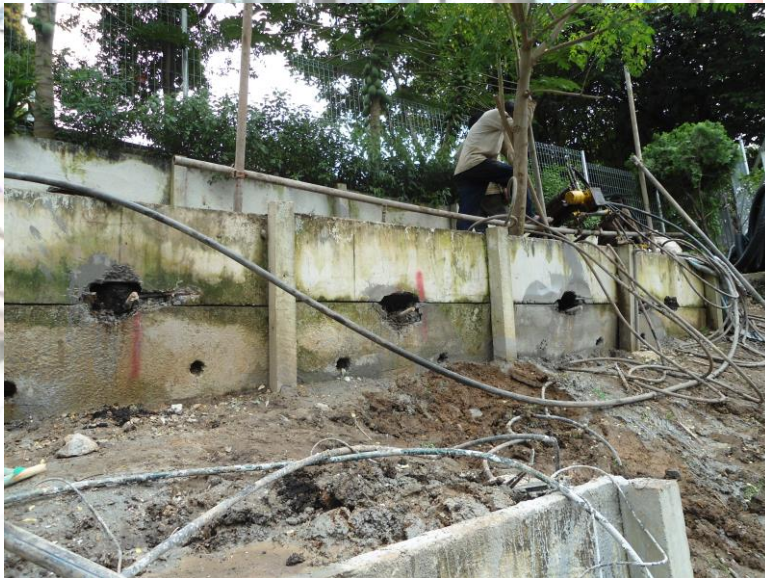
Project : Banglo 3 Tingkat Diatas Lot 3796, No. 48, Jalan Lingkungan Negeri Sembilan Federal Hill, Kuala Lumpur (C02) - Micropiling Works & Soil Nailing Works
