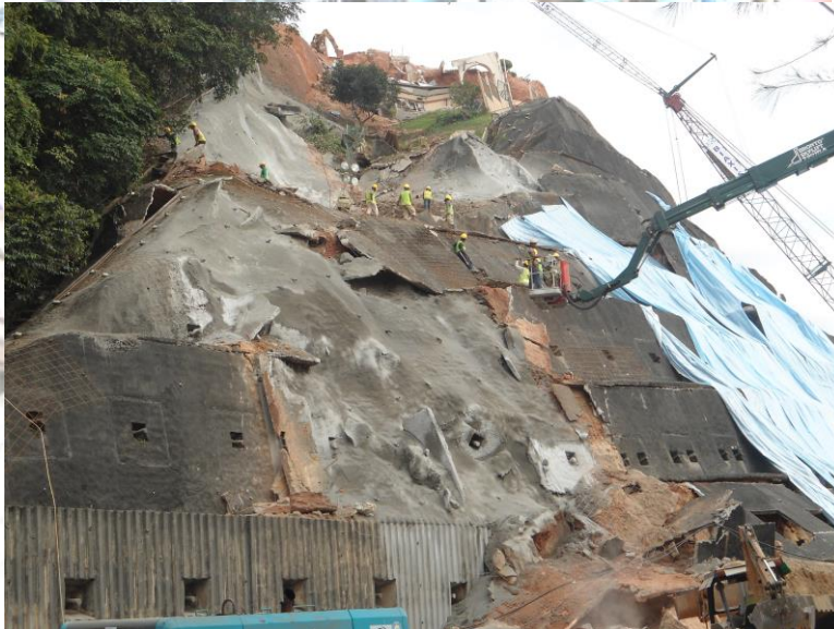
Project : Slope Taman Setiawangsa, Kuala Lumpur - Guniting Works
