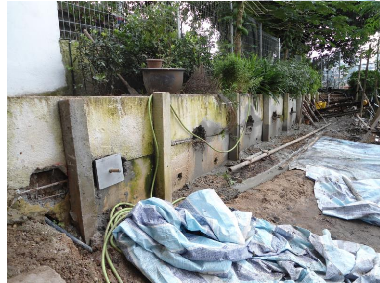
Project : Banglo 3 Tingkat Diatas Lot 3796, No. 48, Jalan Lingkungan Negeri Sembilan Federal Hill, Kuala Lumpur (C02) - Micropiling Works & Soil Nailing Works
