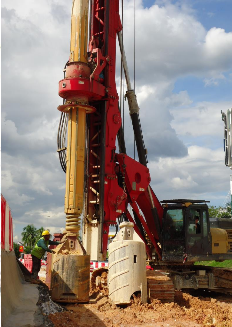
Project : The Construction And Completion of Facilities Works (Package A) For The Kelana Jaya (KLJ) Line Extension Project - Bored Piling Works
