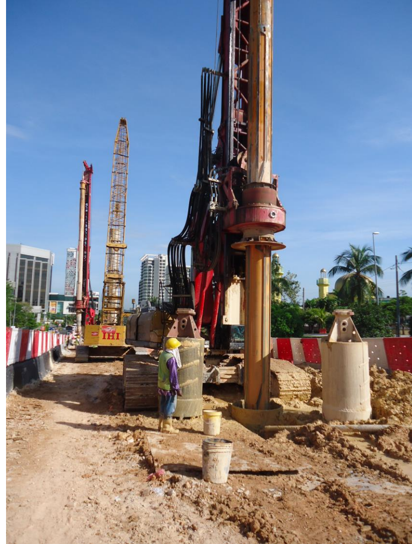
Project : The Construction And Completion of Facilities Works (Package A) For The Kelana Jaya (KLJ) Line Extension Project - Bored Piling Works
