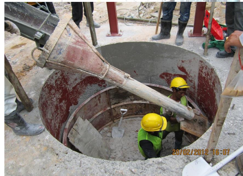
Project : The Construction & Completion of Facilities Works (Package A) For The Kelana Jaya (KJL) Line Extension - Caisson Works
