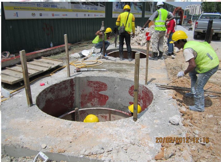
Project : The Construction & Completion of Facilities Works (Package A) For The Kelana Jaya (KJL) Line Extension - Caisson Works
