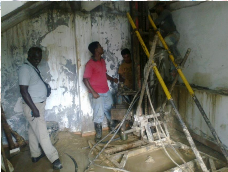
Project : Cadangan Membina 2-1/2 Tingkat Banglo Di Lot 15063, No. 19, Lorong Taman Pantai 1, Taman Pantai, Kuala Lumpur - Underpinning Works
