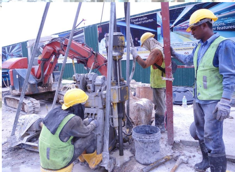
Project : The Construction & Completion of Facilities Works (Package A) For The Kelana Jaya (KJL) Line Extension - Jet Grouting Works
