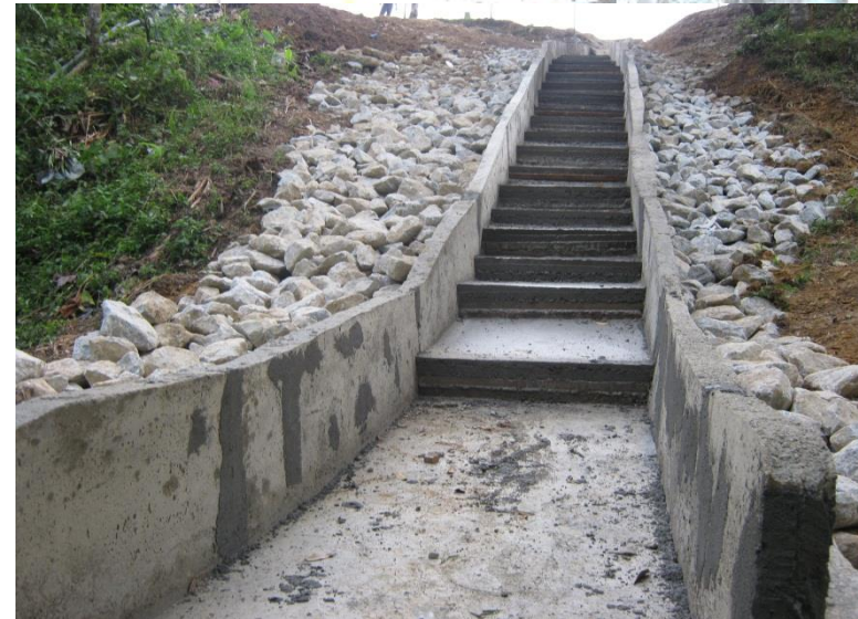
Project : Proposed Repair Works To Slope Failure & Collapsed Cascade Drain At KM 329.55 Northbound, Section C1, North South Expressway - Slope Repair Works
