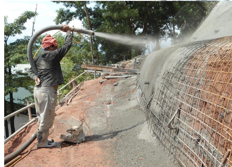
Project : Proposed Slope Strengthening By Soil Nailing With Guniting At Lot 45, Jalan Ehsan Utama, Kawasan Perusahaan Ehsan Jaya, Kepong, 52100 Kuala Lumpur - Slope Strengthening By Soil Nailing With Guniting
