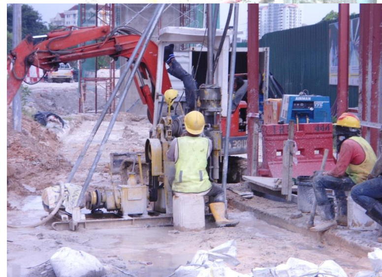
Project : The Construction & Completion of Facilities Works (Package A) For The Kelana Jaya (KJL) Line Extension - Jet Grouting Works
