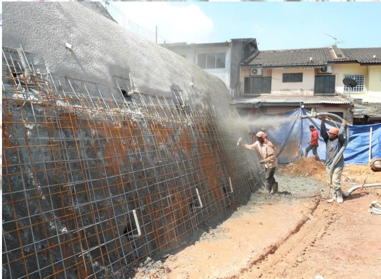
Project : Proposed Slope Strengthening By Soil Nailing With Guniting At Lot 45, Jalan Ehsan Utama, Kawasan Perusahaan Ehsan Jaya, Kepong, 52100 Kuala Lumpur - Slope Strengthening By Soil Nailing With Guniting
