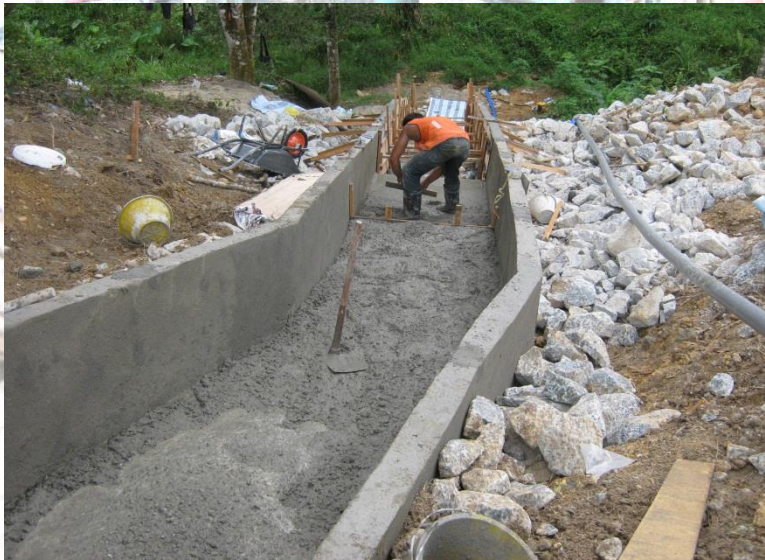
Project : Proposed Repair Works To Slope Failure & Collapsed Cascade Drain At KM 329.55 Northbound, Section C1, North South Expressway - Slope Repair Works
