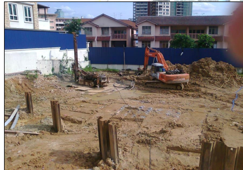
Project : Cadangan Membina 2-1/2 Tingkat Banglo Di Lot 15063, No. 19, Lorong Taman Pantai 1, Taman Pantai, Kuala Lumpur - Preboring Works For RC Pile Works
