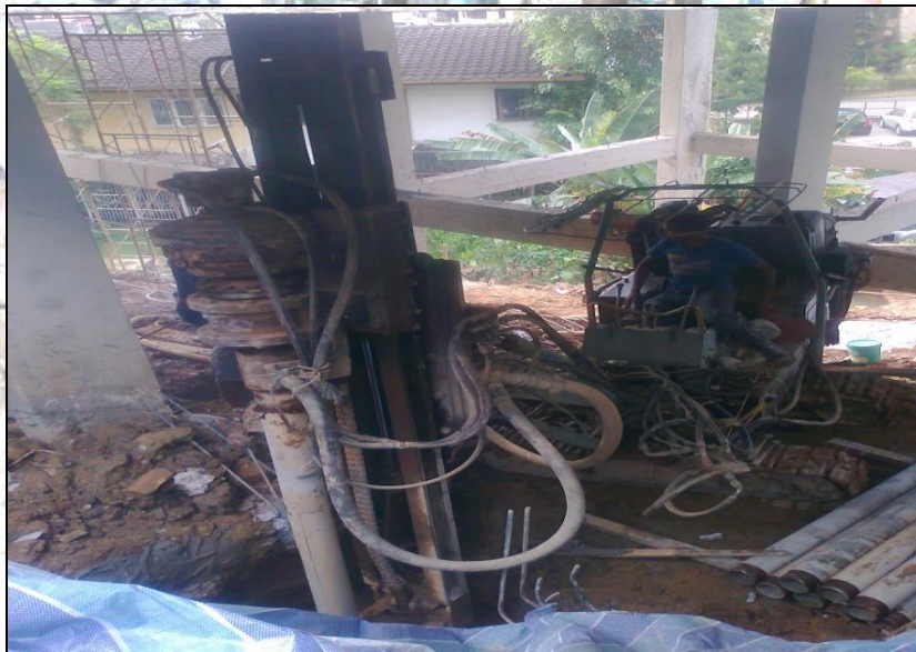
Project : Banglo 3 Tingkat Diatas Lot 3796, No. 48, Jalan Lingkungan Negeri Sembilan Federal Hill, Kuala Lumpur - Underpinning By Micropiling Works
