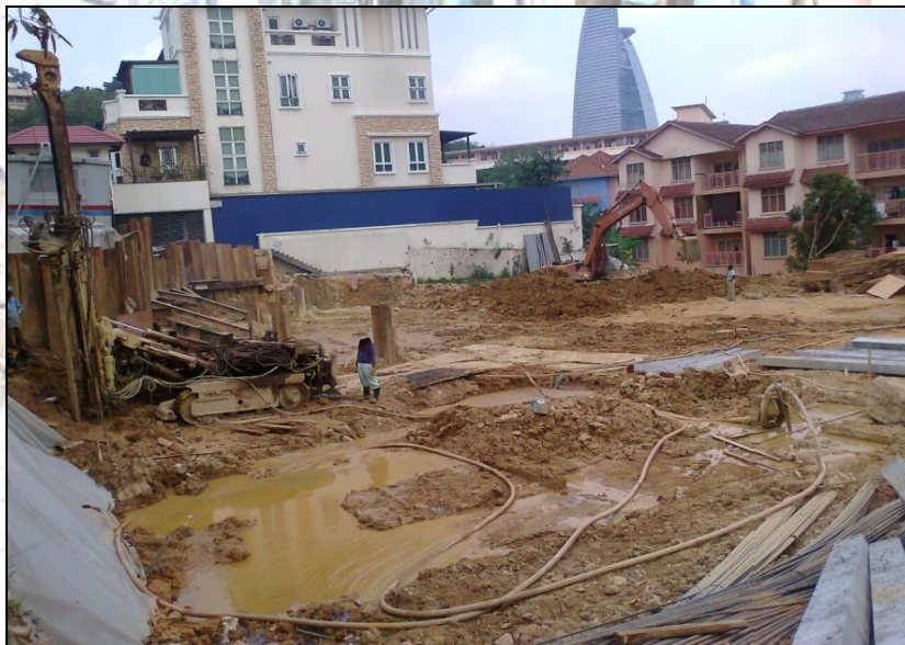
Project : Cadangan Membina 2-1/2 Tingkat Banglo Di Lot 15063, No. 19, Lorong Taman Pantai 1, Taman Pantai, Kuala Lumpur - Preboring Works For RC Pile Works
