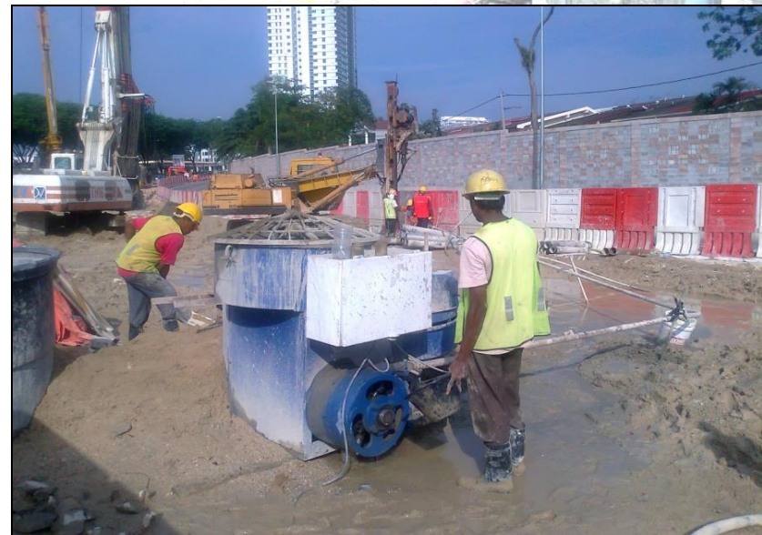
Project : Proposed Upgrading For Taman Tun Dr. Ismail Interchange At Lebuhraya Damansara-Puchong (LPD4) - Cement Sand Grout Column
