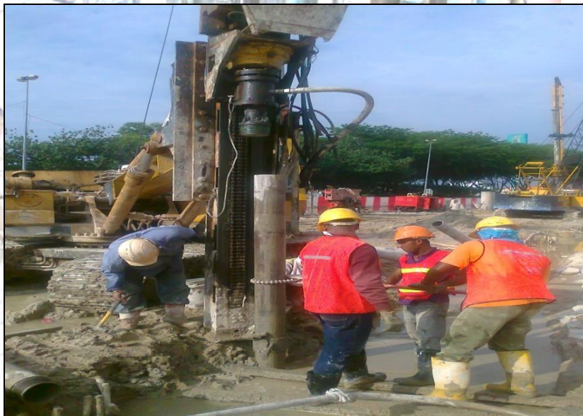
Project : Proposed Upgrading For Taman Tun Dr. Ismail Interchange At Lebuhraya Damansara-Puchong (LPD4) - Cement Sand Grout Column
