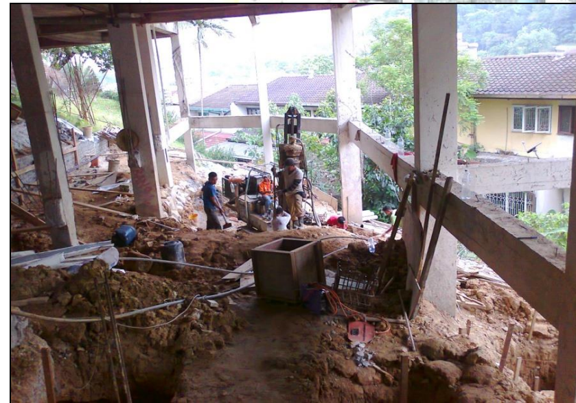
Project : Banglo 3 Tingkat Diatas Lot 3796, No. 48, Jalan Lingkungan Negeri Sembilan Federal Hill, Kuala Lumpur - Underpinning By Micropiling Works
