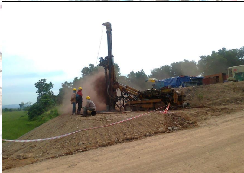
Project : Kolej Pertanian Malaysia (KPM), Bukit Tangga, Kedah Darul Aman - Micropiling Works
