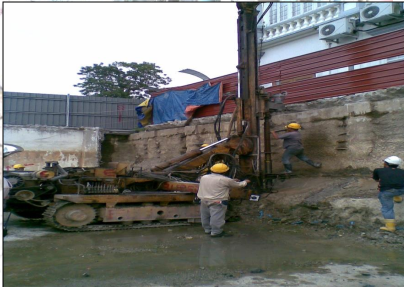
Project : Plaza Merdeka Kuching Commercial Complex / Hotel, At Pearl Street, Kuching, Sarawak - Micropiling Works
