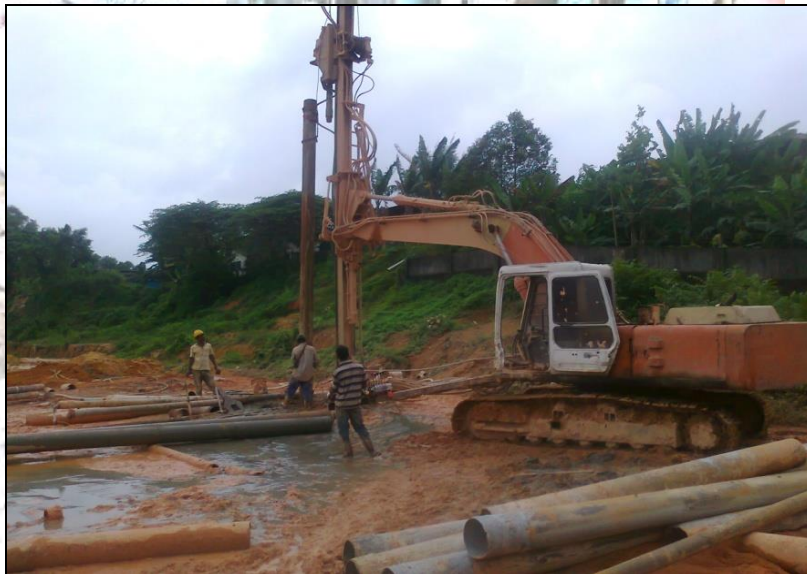
Project : Pusat Pertahanan Awam, Kuantan, Pahang - Micropiling Works
