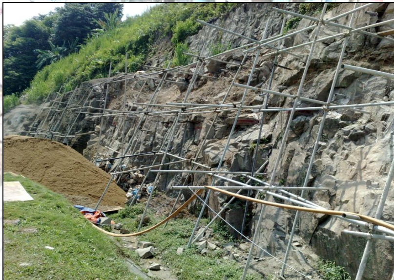
Project : Proposed Remedial Works For Rock Slope At West Bound, Section C4, JalanDamansara Toll - NKVE - Guniting Works
