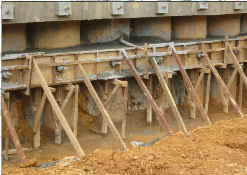
Project : Electrified Double Track Project Between Seremban & Gemas - Soil Nail Concrete Grid Beam At CBP Wall
